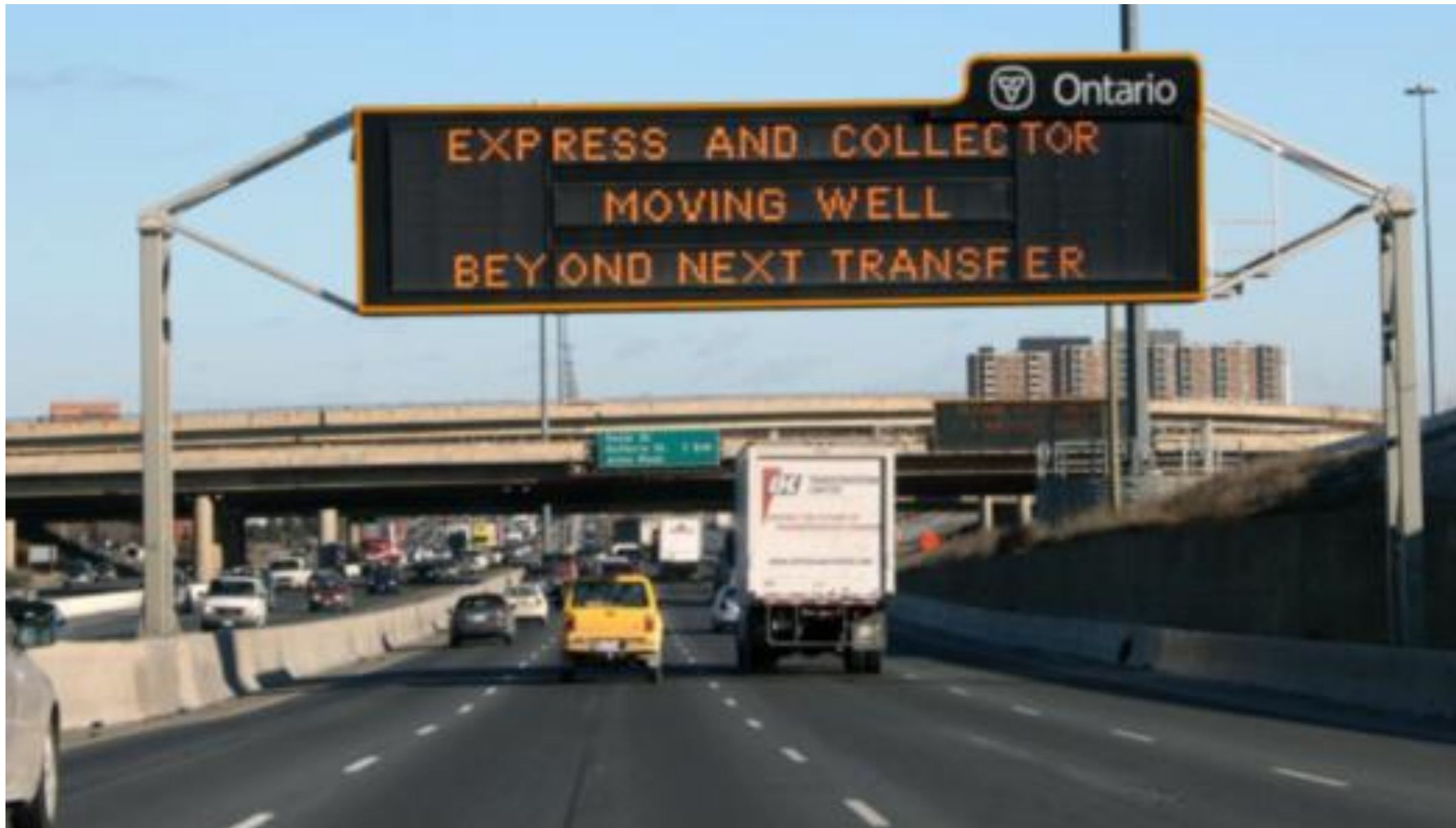
Intelligent Transportation Systems Features (variable message signs, real time traveler information)
